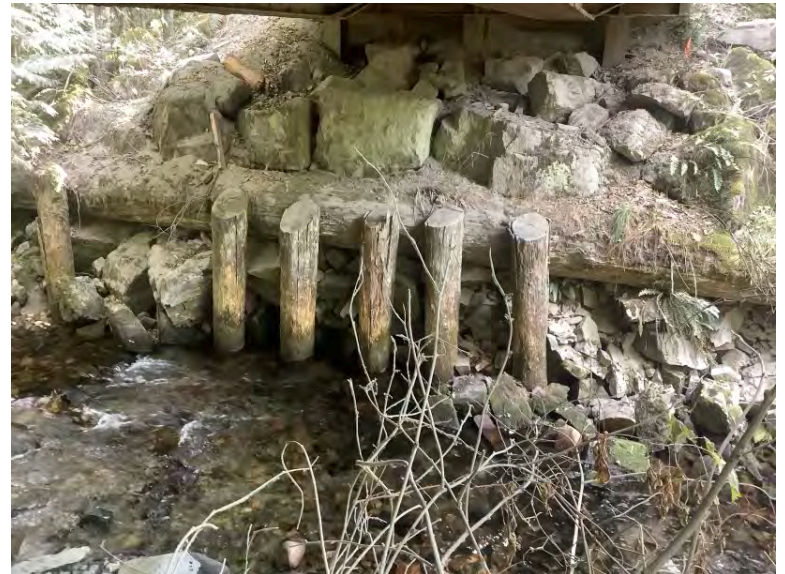
Right Bank Abutment when facing downstream
